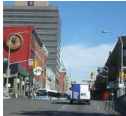
South gateway approaching on Richmond Street
